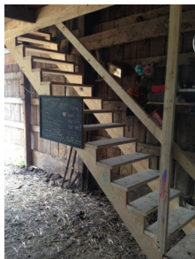
Site built wood stairs
